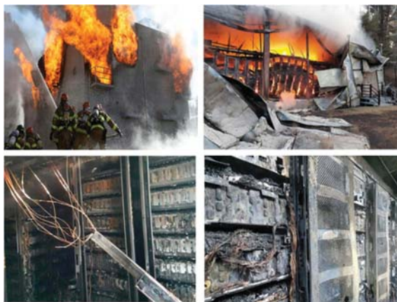
Figure 14: Fire Damage at Korean BESS Facilities 229
